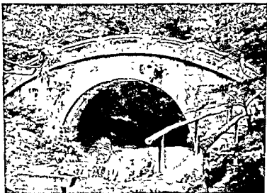
Stone-bridge in Kōraku-en, Tokyo
